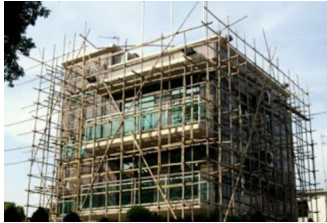
Plate 2.2 bamboo used for scaffolding in Nigeria (Anon.2015)
