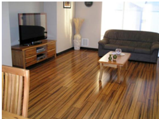
Plate 2.3 Bamboo flooring system in Nigeria (Anon 2015)
