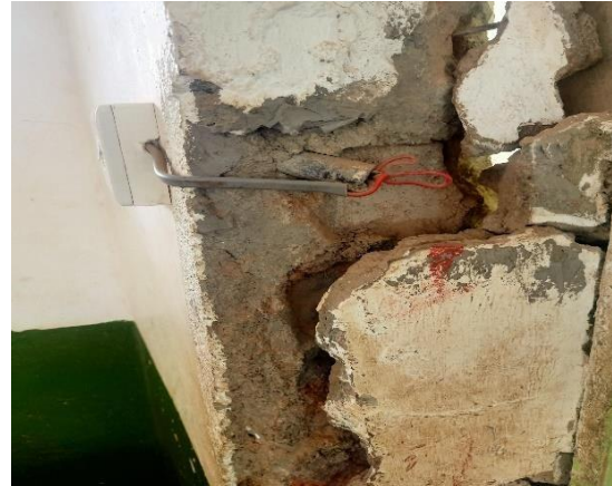
Plate 5.2: Electrical switch in a class
