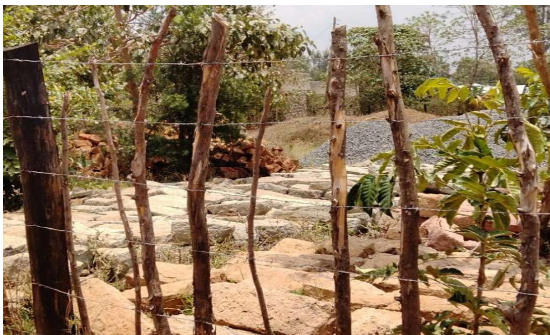
Plate 5: Blocks and ballast for construction
