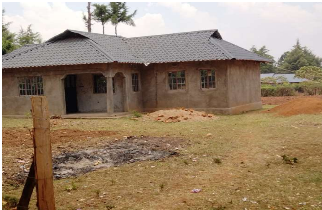
Plate 4: Residential house under construction
