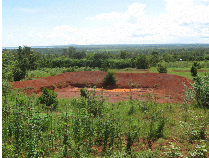
Plate 3 Water-pan under construction (Lower RNB)
